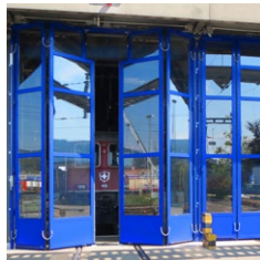
Railway Depot Doors
